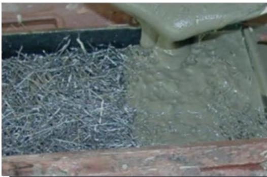
Figure 1. Casting procedure of SIFCON
