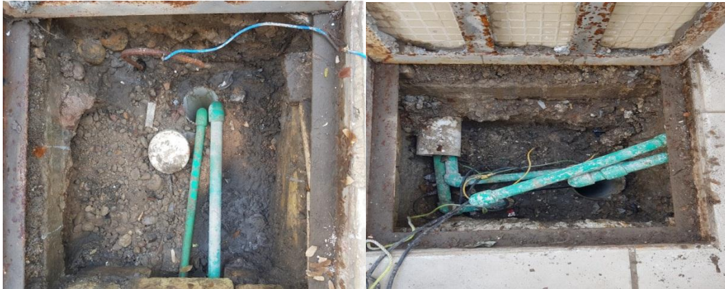
Figure (2): The Source and drain holes.
