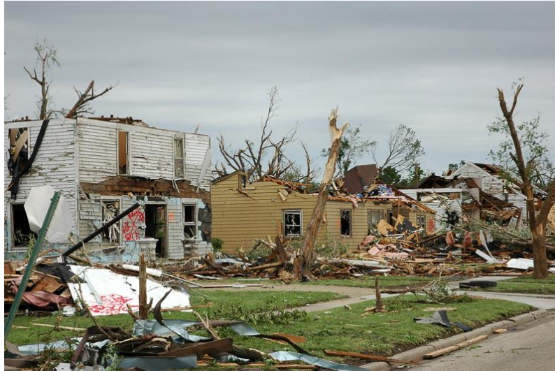
Figure (1). Massive destruction of trees and buildings due to windstorm.
