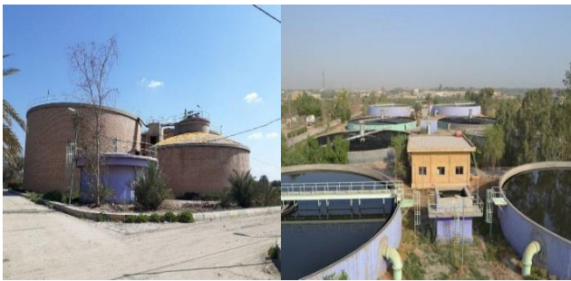
Figure 1. A sewage treatment plant in Al Kufa city [6]
