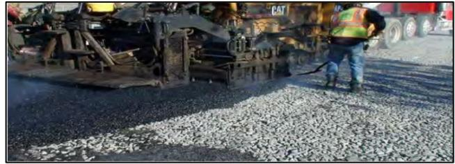
**Figure 3.** Porous asphalt paving [45]
