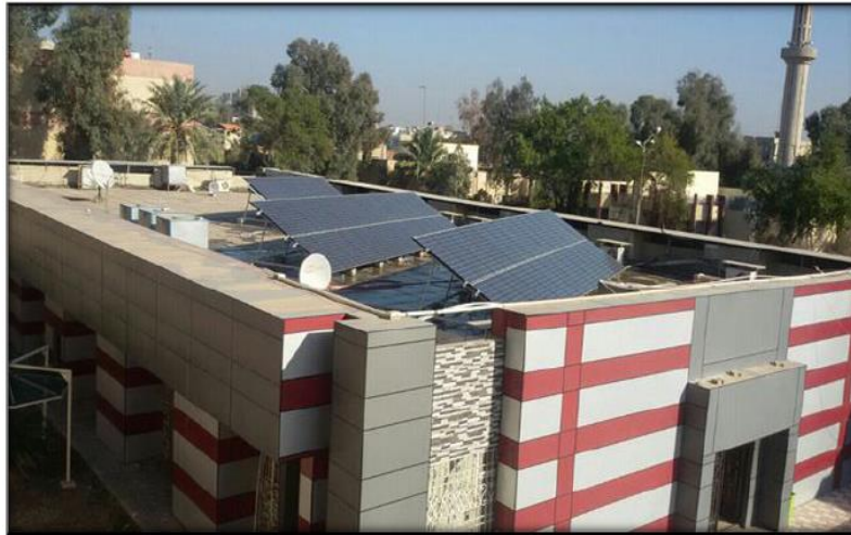
. Figure . 1. 15kW solar PV system.
