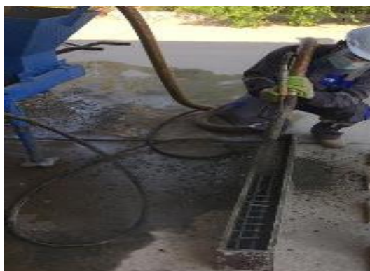
Figure .4 Shotcrete concrete casting process
