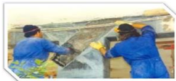
Figure 3 Reinforcement of joints [14]
