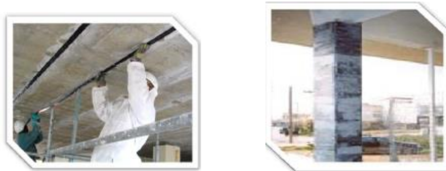
Figure 2 Reinforcing Slabs, Beams, and Columns [14]
