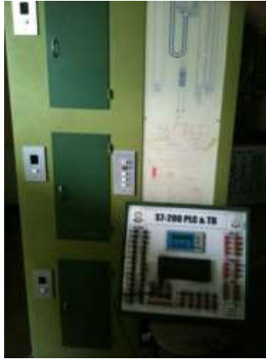
Fig. 21 The Didactic Elevator after Rehabilitation
