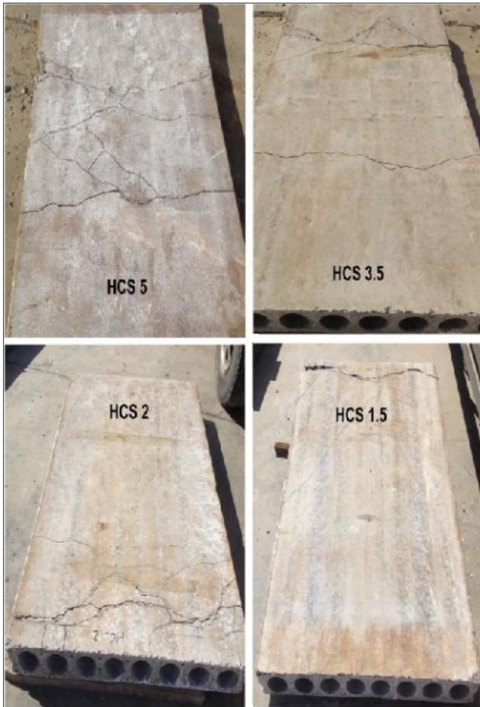
Figure 4. Cracks pattern at the tension surface of the four specimens.
