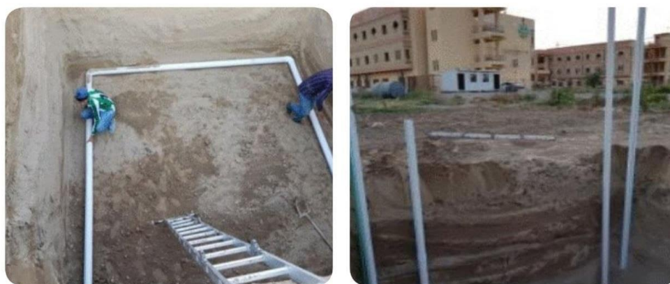
Figure 4 Earth- air heat exchanger
