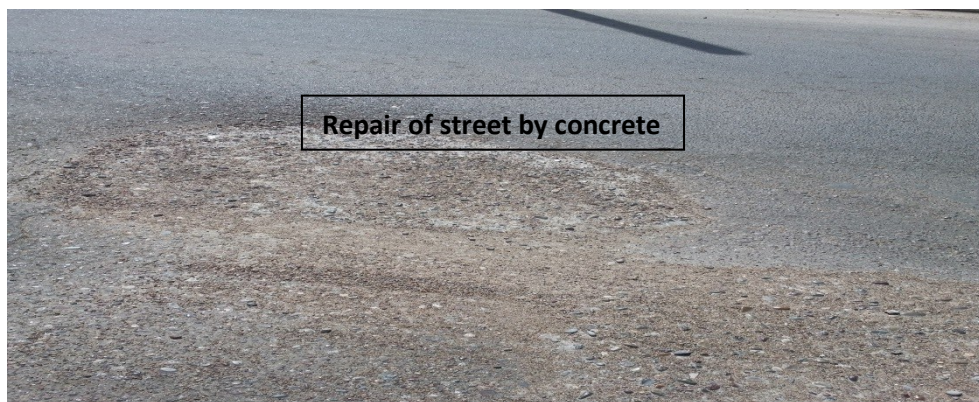
Plate 5 (B) Repair of upper layer of street by concentrate
