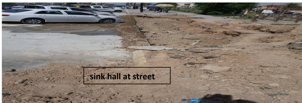
Plate 2 (B) Sink hall in Major Street near Passports office
