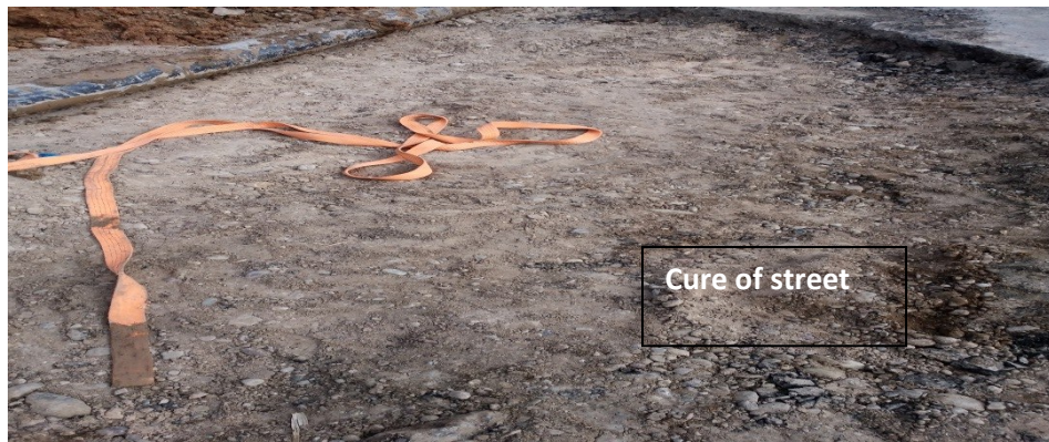
Plate 5 (A) Exchange layer of street for repair it
