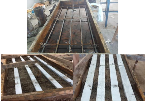
Figure 4. Steel reinforcement and polystyrene foam
