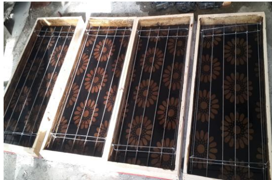
Figure (1) Steel reinforcement cage and formworks
