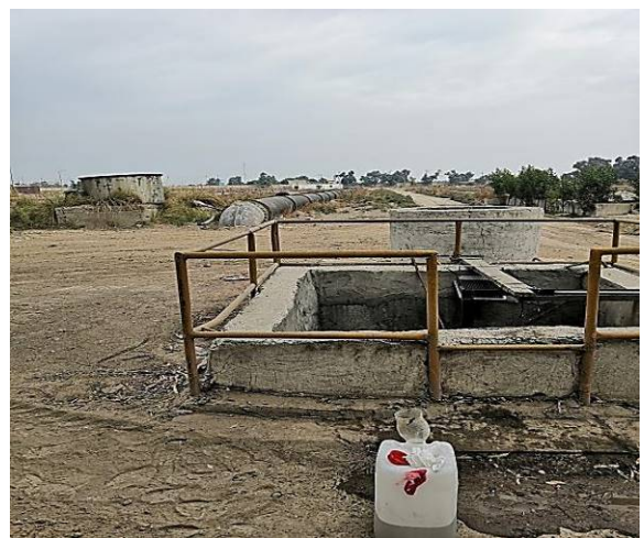
Figure 3. Crude wastewater intake basin
