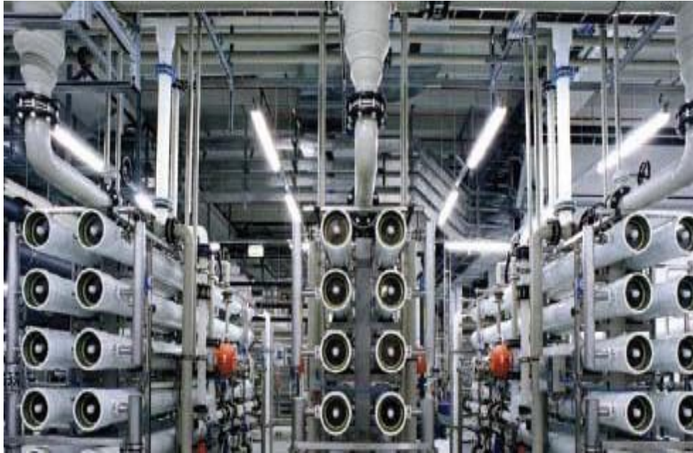
Fig.5: The Cell and Stages of Water Treatment Unit in Thermal Power Station
