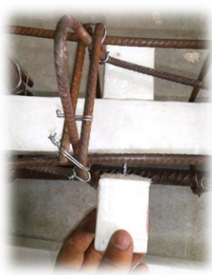
Fig (5): Preparing the Opening Mold (Top View)
