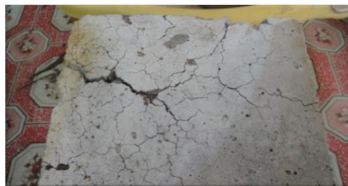
Figure 6. The surface of the cub with GL51 after 3 hr fire
