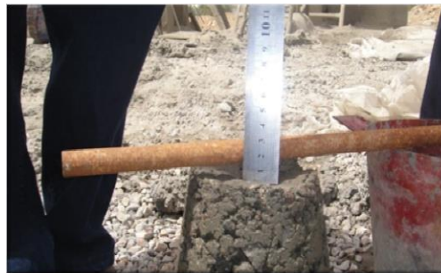
Figure 1. The fresh concrete without GL51 gives a slump test of 30mm
