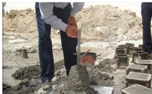
Figure 2. The fresh concrete with GL51( 1L/m3) gives a slump test of 90mm
