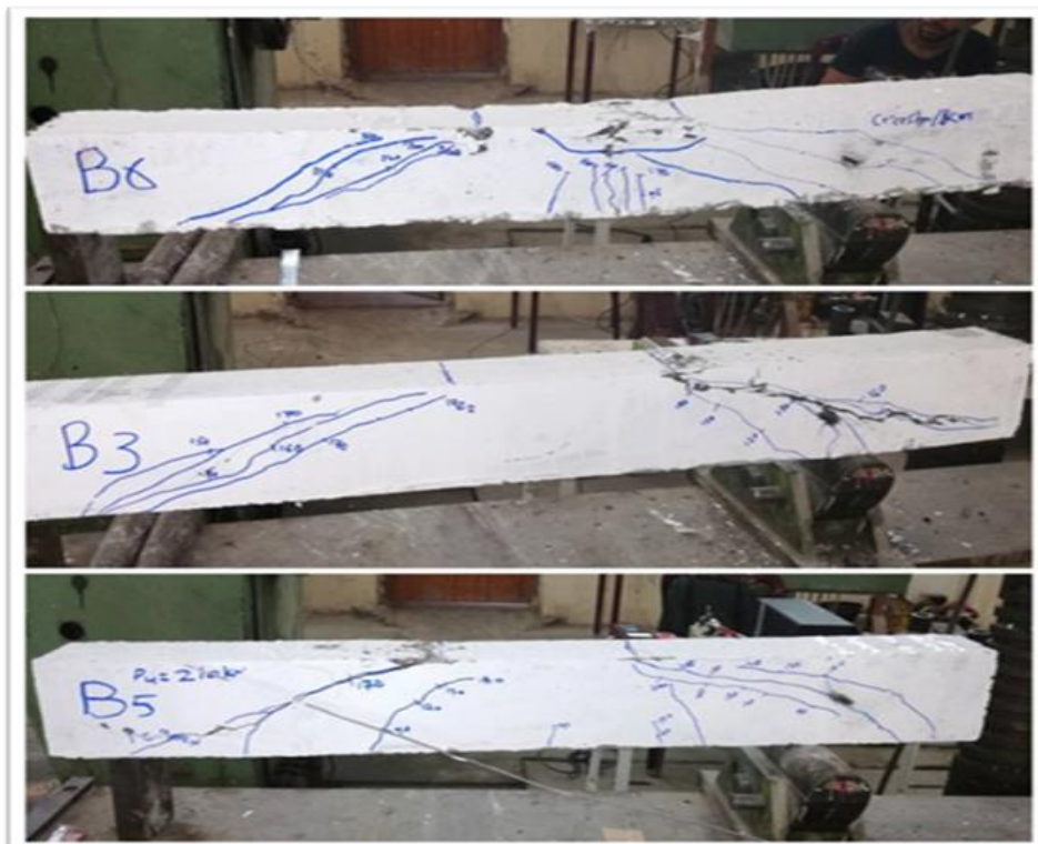
Plate (3) Crack Pattern of Beams
