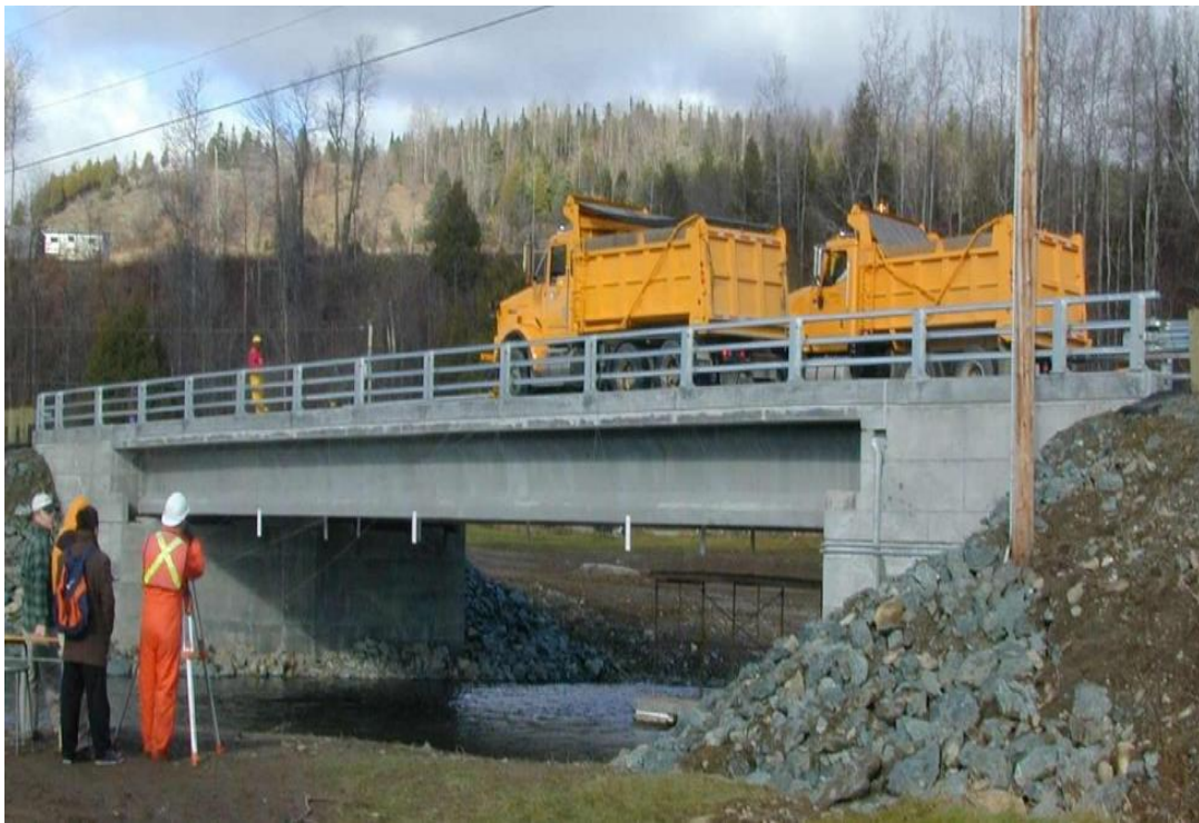
(a)Wotton Bridge, Canada.
