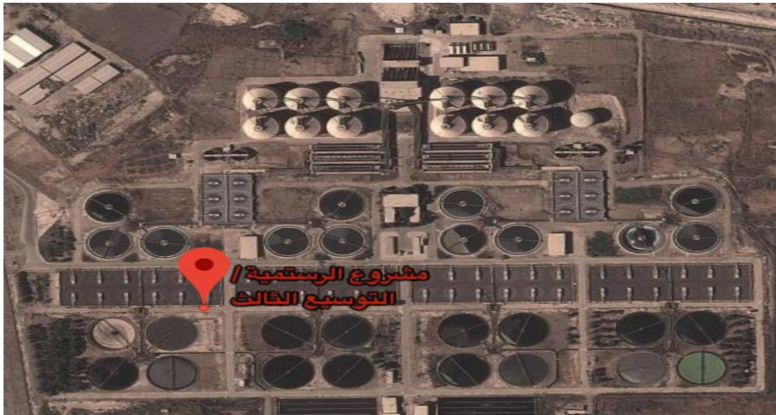
Figure 3. Show Northern Rustimeh WWTP from the Top [8].
