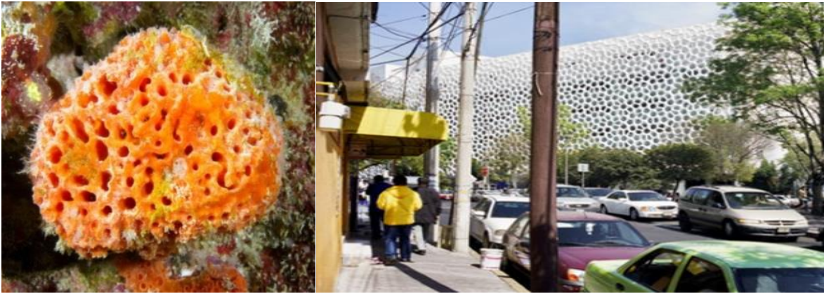
Figure 4: The Torre de Especialidades facade at the Hospital of Manuel Gea Gonzalez
