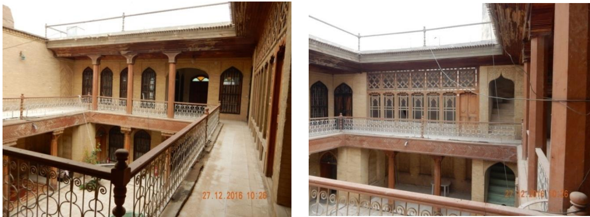
Figure 3. Examples of traditional Baghdadi house showing the courtyard (hosh) and tarma (colonnade veranda).
