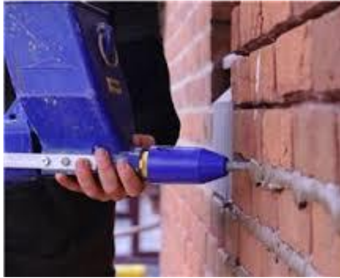
Figure 9. Repointing process using cement mortar in a brick wall.
