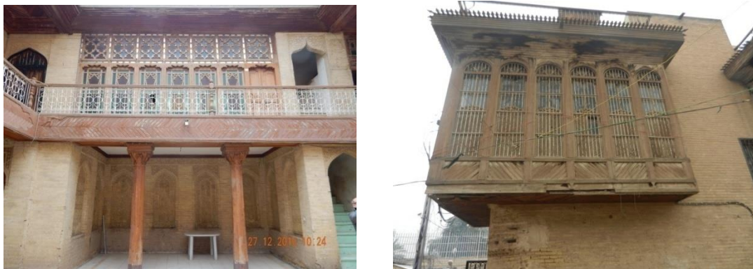
Figure 4. Examples of talar in Baghdadi house (left) shanashil landed into the street (right)
