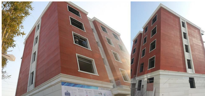
Figure 9. 3D printed Five-story apartment in China [30]
