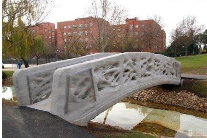
Figure 12. 3D printed Concrete Bridge in Spain [40]
