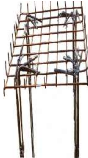
Plate 2: Reinforcement of the pile groups.
