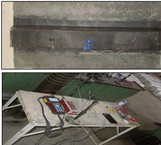
Figure 6. Data logger and location of strain gauges
