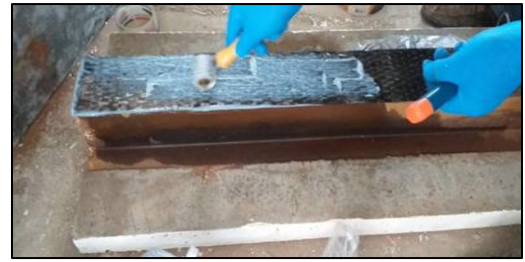
Figure 5. Strengthening of corroded bottom flange by CFRP Strip
