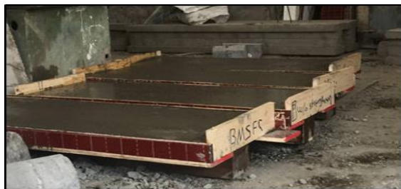
Figure 2. Beam Specimen Deck Slab Cast
