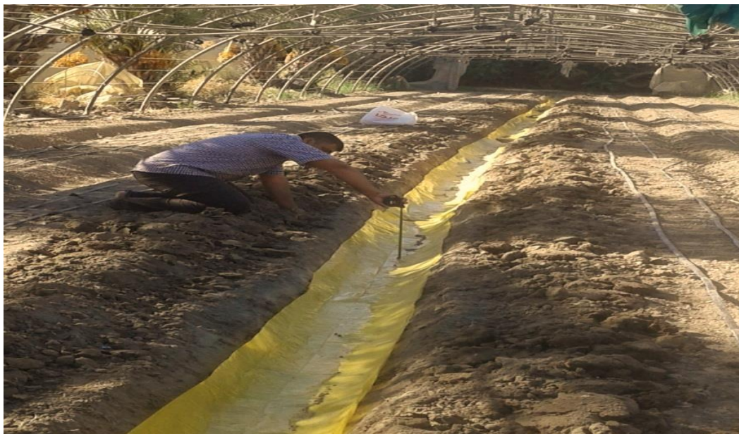
Figure (3) Installation of the polyethylene sheet below the soil surface.
