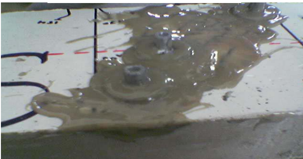
Fig. (3): Epoxy Injection Process
