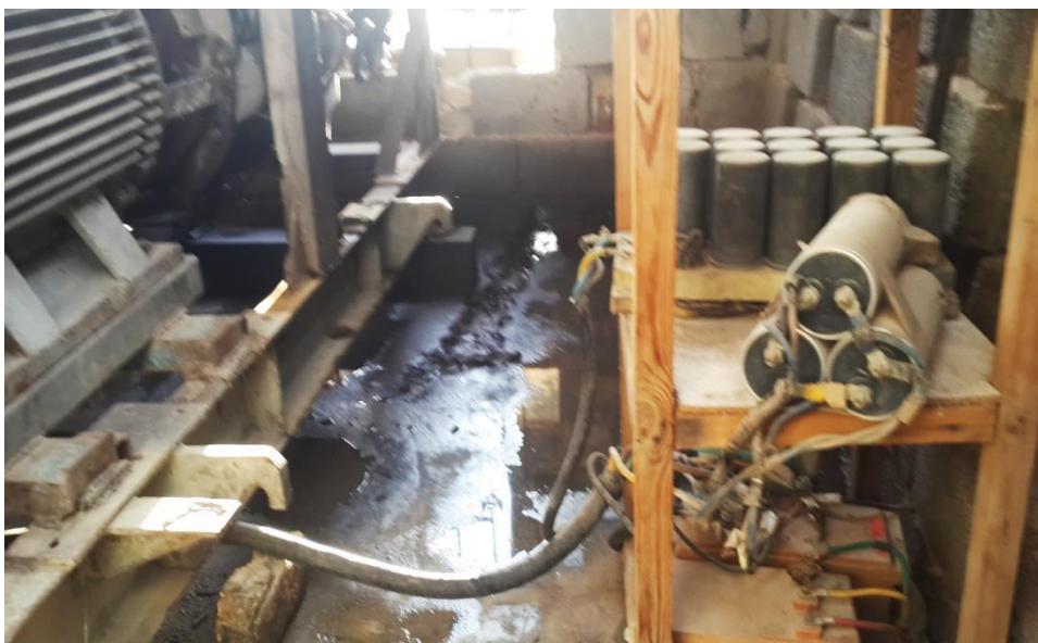
Fig.4 Show the connection between the induction generator and the capacitors
