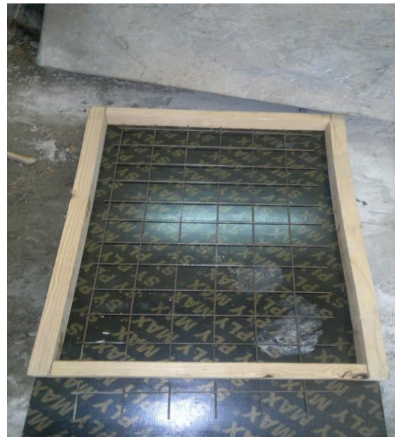
b) steel reinforcement
