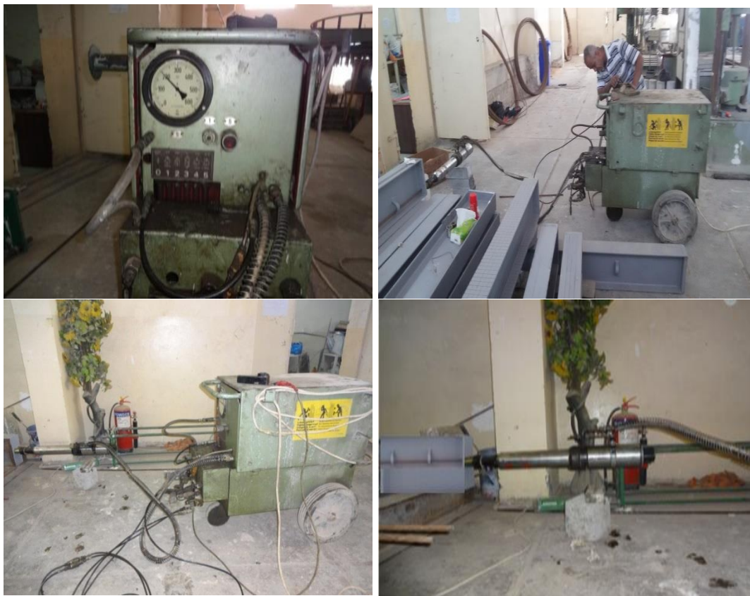
Figure (6) Hydraulic machine and single strand jack prestressing strand.
