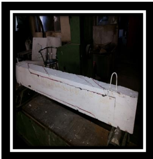
Figure (14): Crack Pattern and Failure Mode of Composite beam (B2)
