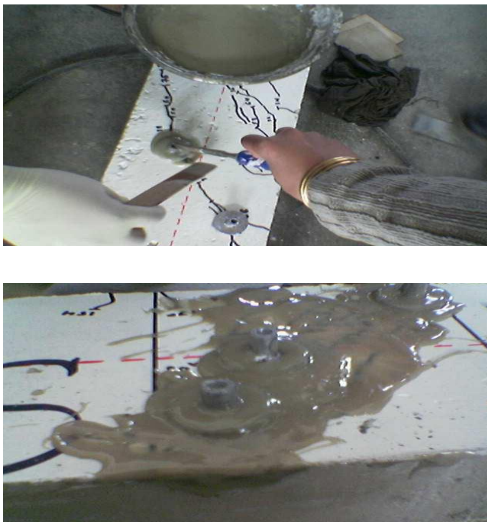
Fig. 3 . Epoxy Injection Process
