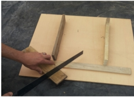
a) preparation the framework for the Concrete retaining wall.
