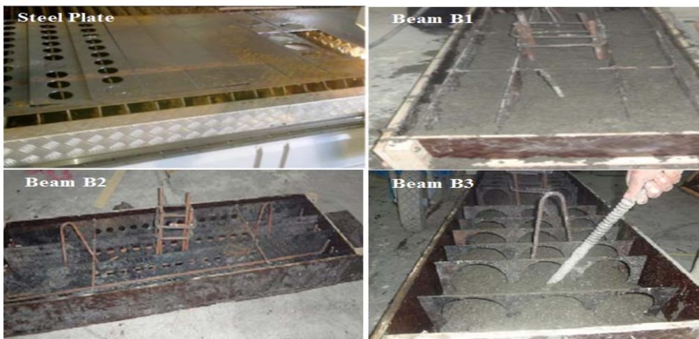
Figure (2) Gagger steel plate used in B1, B2 and B3
