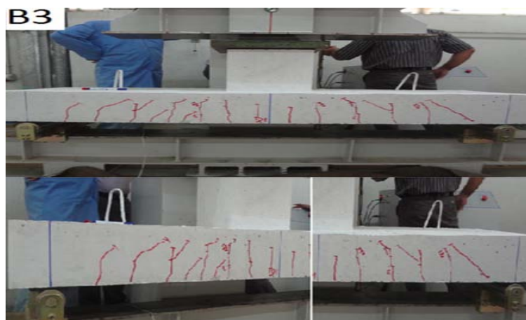
Figure (9) Crack pattern for (B3)
