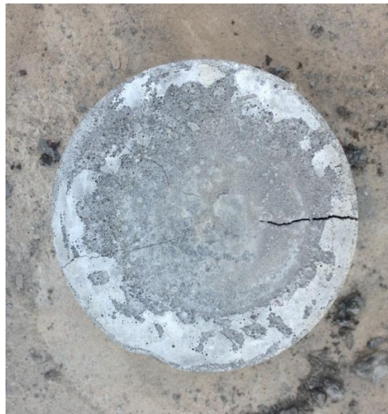
Fig .(10) First crack for cylindrical specimen mixture C5
