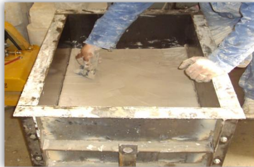
Plate No. (5): Leveling of the Top Layer.
