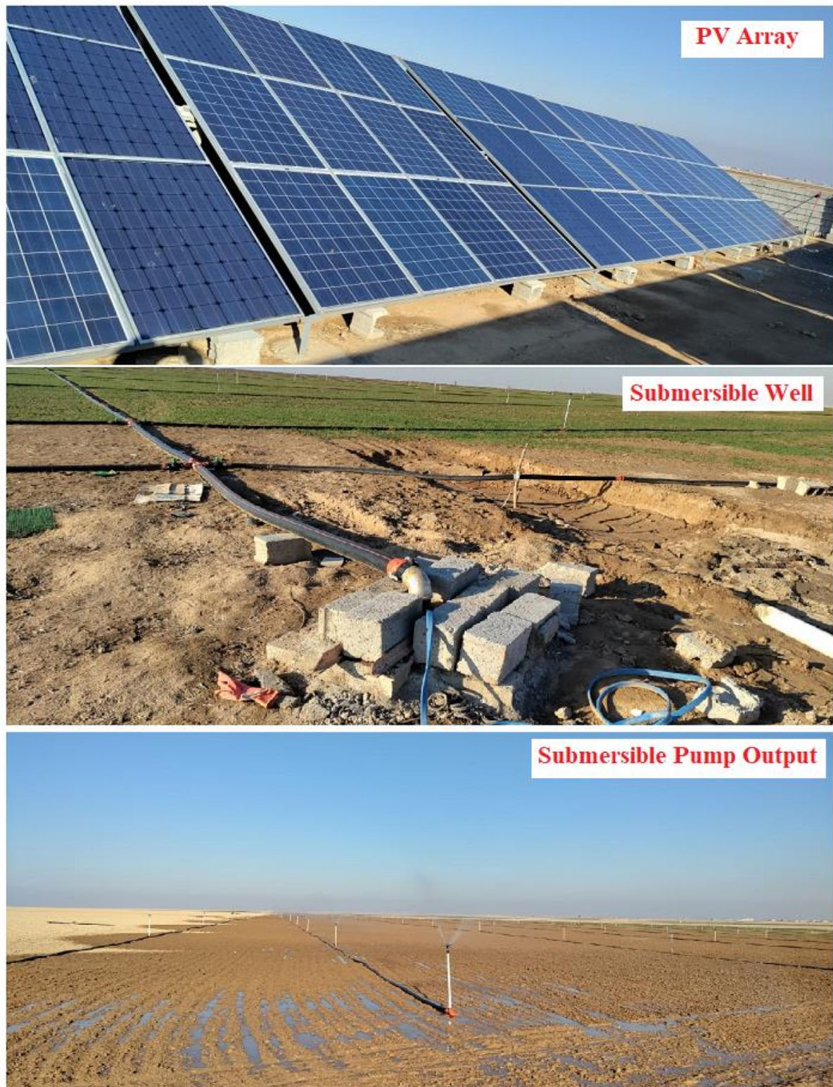
Fig. 20 The Installed PV Array (Top), Submersible ACIM Pump (Middle), and the Field to be Irrigated by the System (Bottom).
