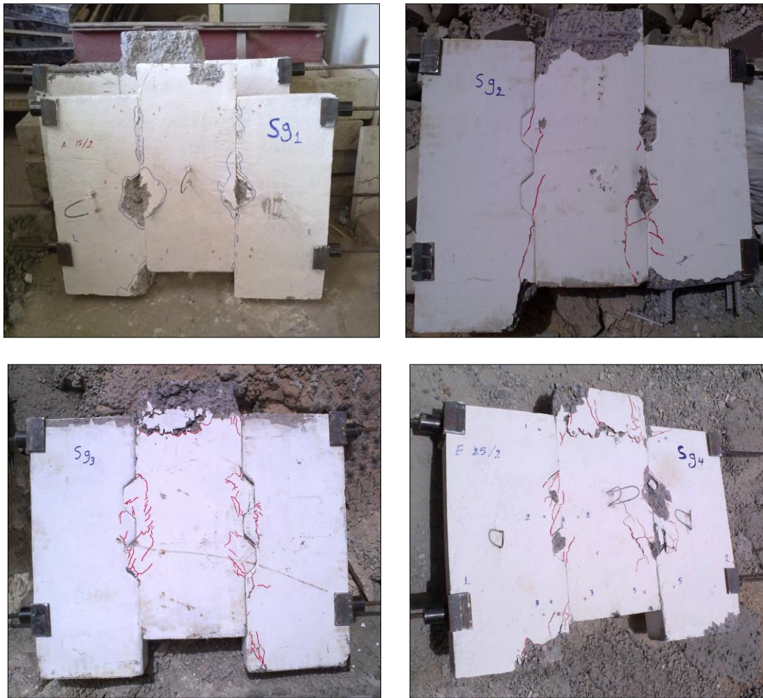
Figure (6)-(A)- Crack Pattern of Tested Specimens
