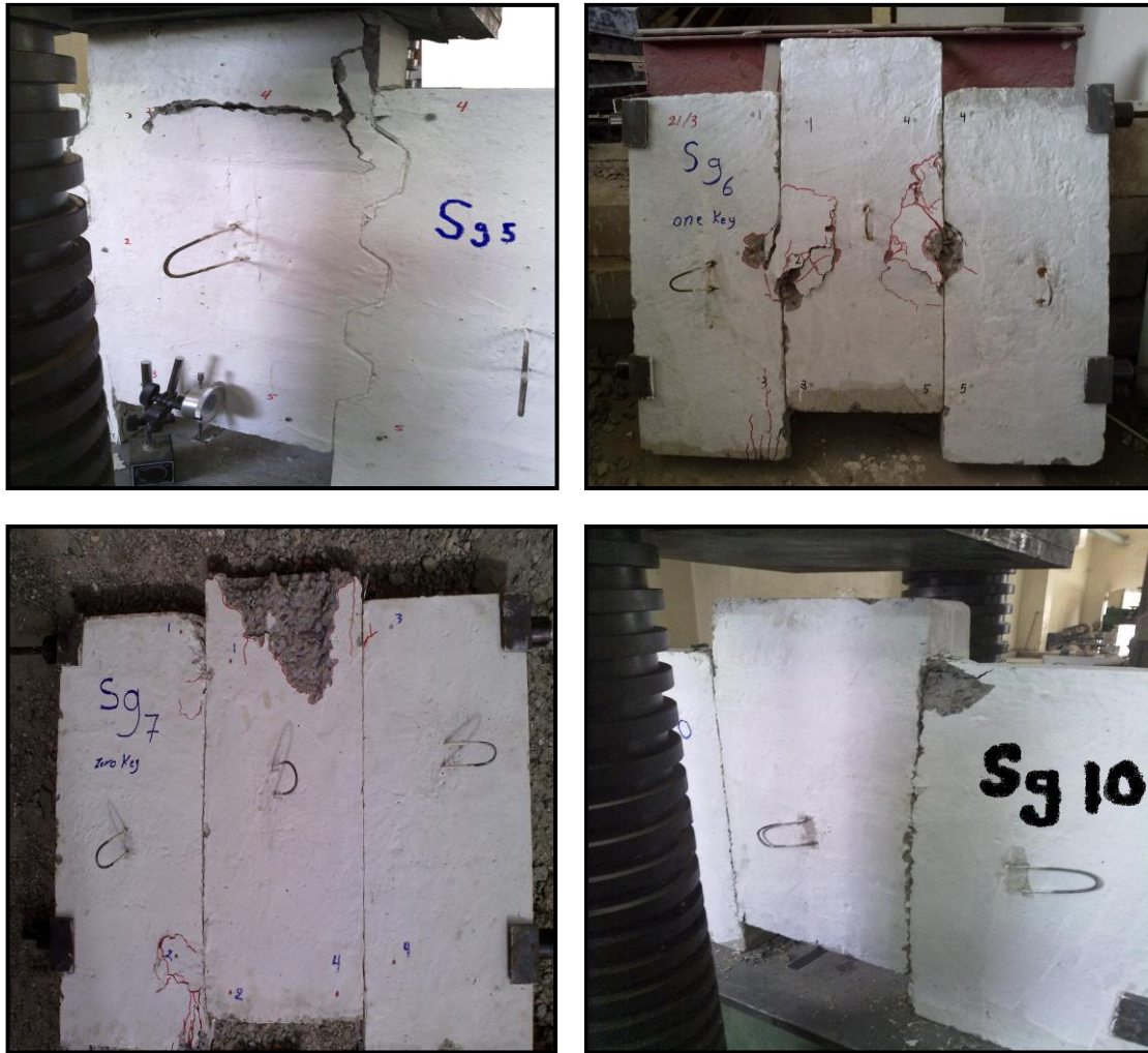
Figure (6)-(B)- Crack Pattern of Tested Specimens (Continue)
