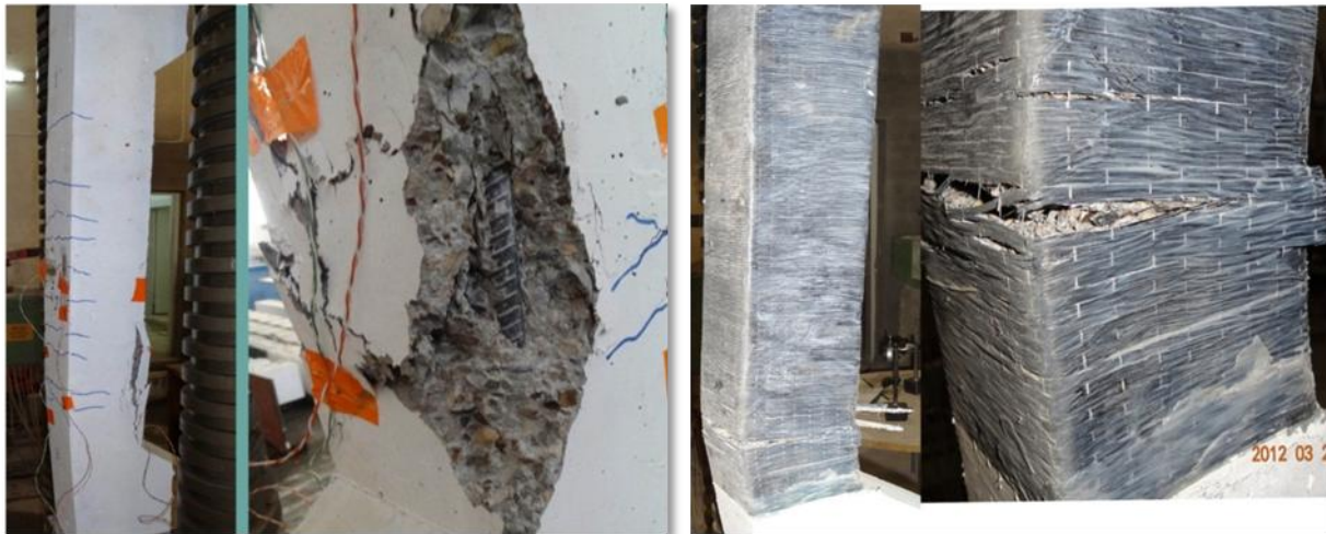
Figure (12) Crack pattern for column.
