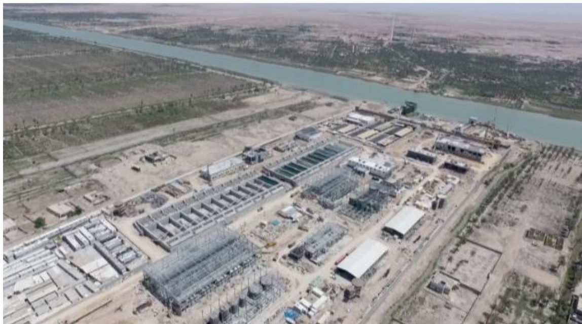
Figure 1. Aerial view of JICA assisted Water Treatment Project in Hartha, Basrah, Iraq.
