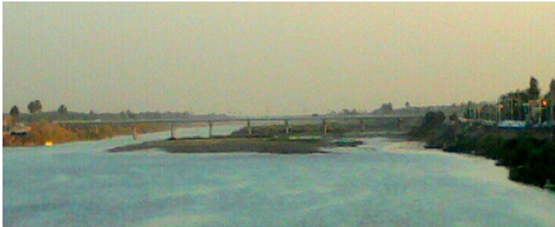
Figure (2): Al- Hindiya second bridge
