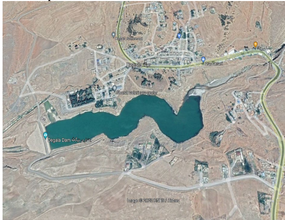
Fig. 1 Degala Dam View.
