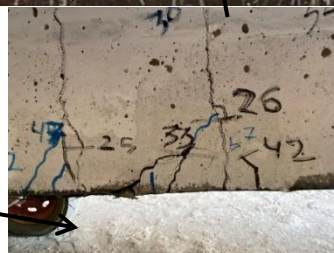
Fig. 10 Failure in HCS-R100 Specimen.
