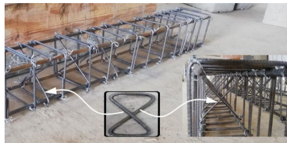
Plate 1 Internal Cross-Rod Steel Reinforcement Details.
