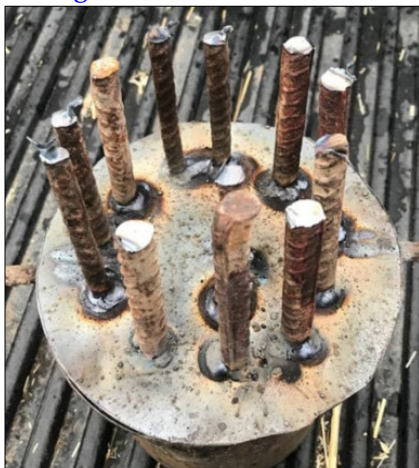
Fig. 2 Steel Bars Connected with Copper Wire.
