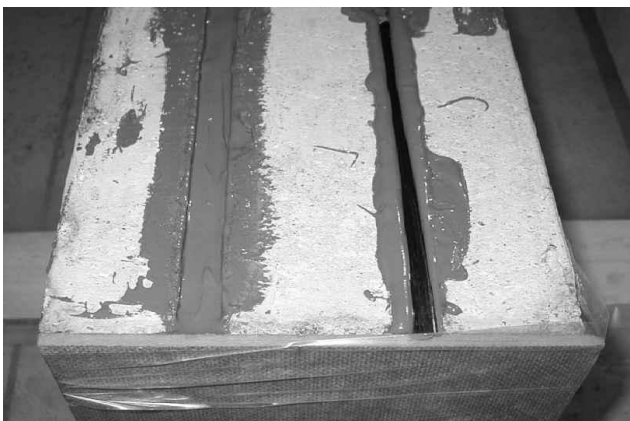
Fig.2 10 mm square rods bonded in slots in the concrete cover
