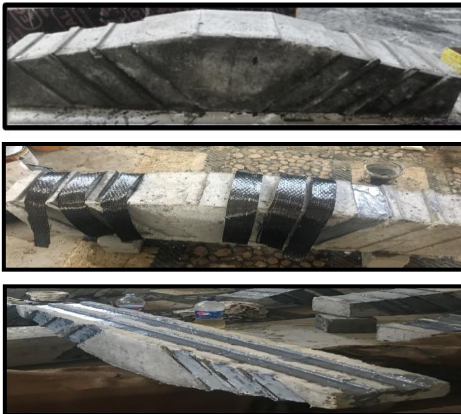
Plate 3. Process of the CFRP installation in the grooves.
