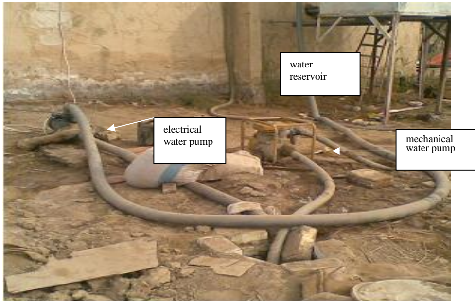
Figure (1): A photograph represents the artesian well used for the processing of hatchery water.
