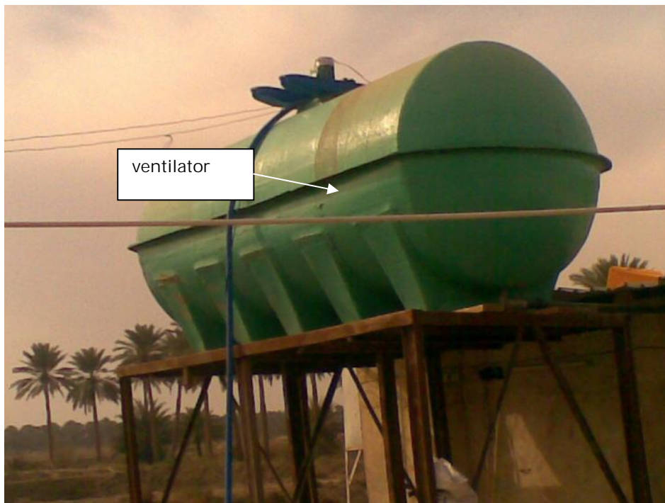
Figure (2): a photograph represent the main reservoir for water and Ventilator.
