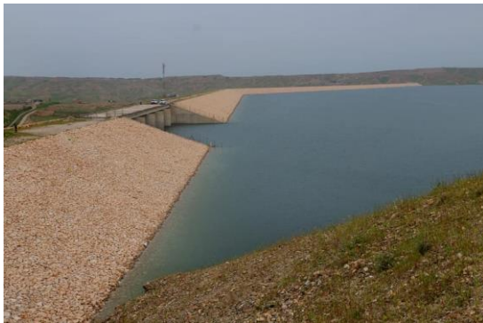
Figure 1. Khassa Chai dam
